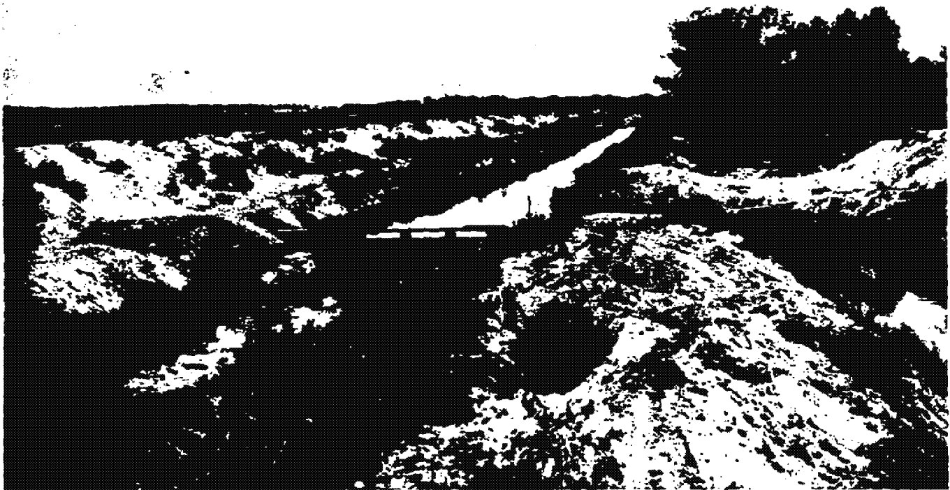
FIGURE 19.—Riverside drain in Middle Rio Grande Conservancy District, New Mexico. Check structure diverts water into canal for irrigation.
